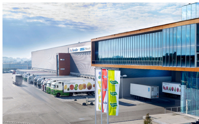
The Greenery has a fully automated logistical infrastructure.
